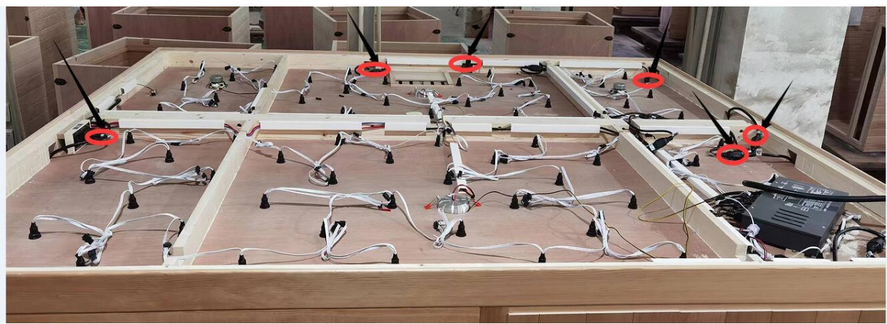
Figure 19 Connect All (6) Of The Heater Cord Connections
