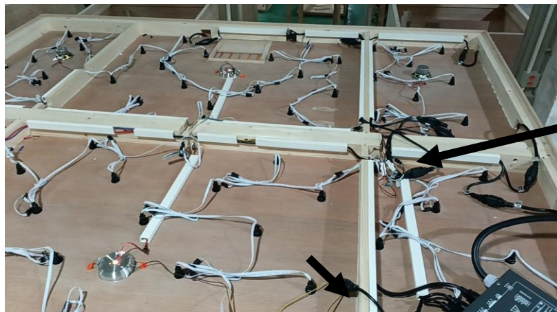
Figure 18 Harness & Speaker Connections
